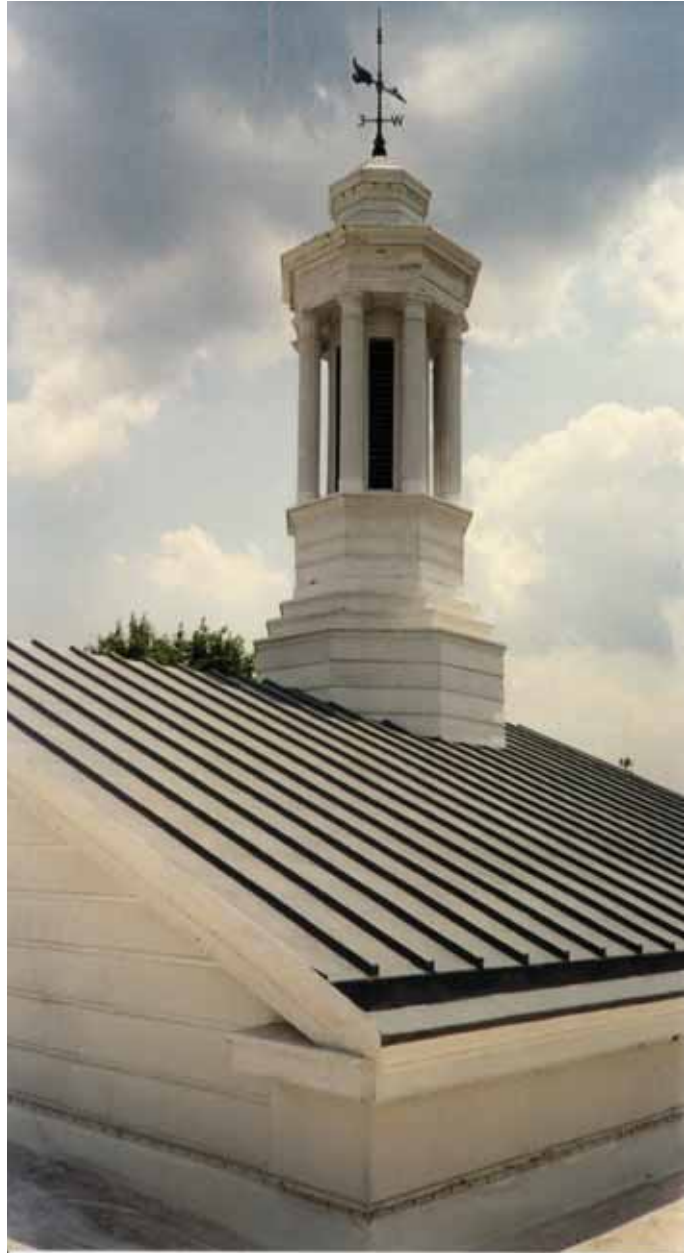
Cupola and recently restored tin roof
