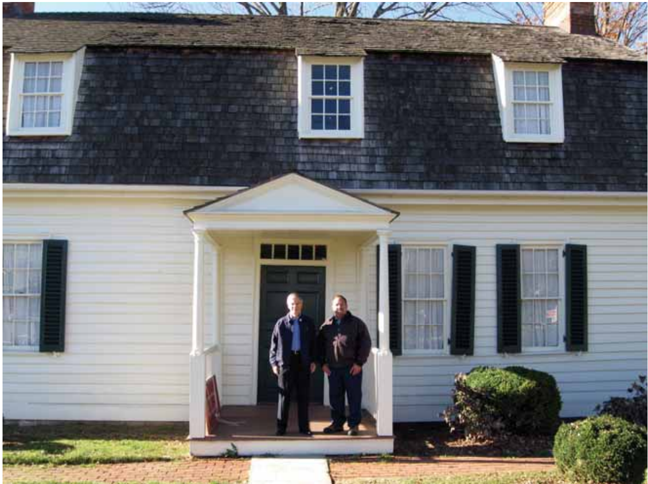
The Hays House after renovations
